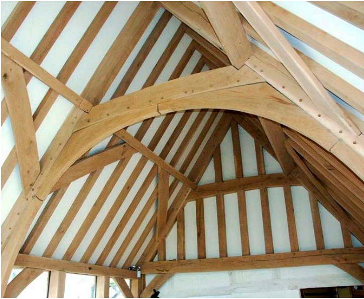
Arched brace collar truss
